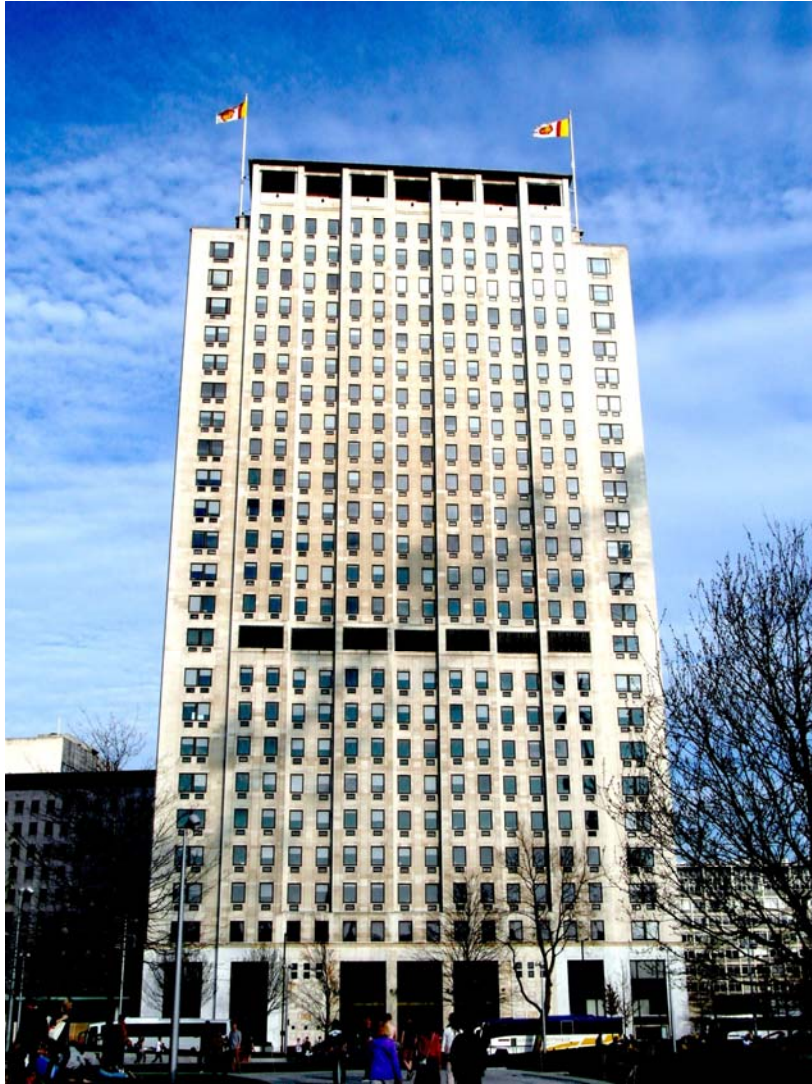
The Shell Centre headquarters in London, 2019. (Reading Tom, Wikimedia Commons, CC BY 2.0)
