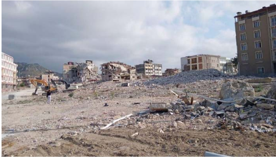
Earthquake damage in Hatay, Turkey, December 2023 January 2024
