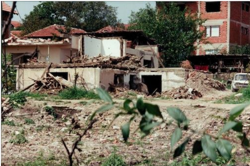
Damaged home near bombed neighborhood of Nishka and Uzhička Streets. Photo: Gregory Elich.
