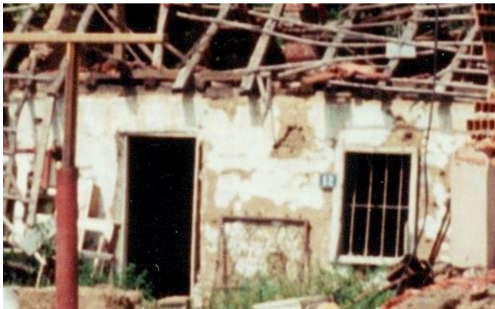
Damaged home adjacent to destroyed neighborhood on Vuk Karadzich Street. Photo: Gregory Elich.
