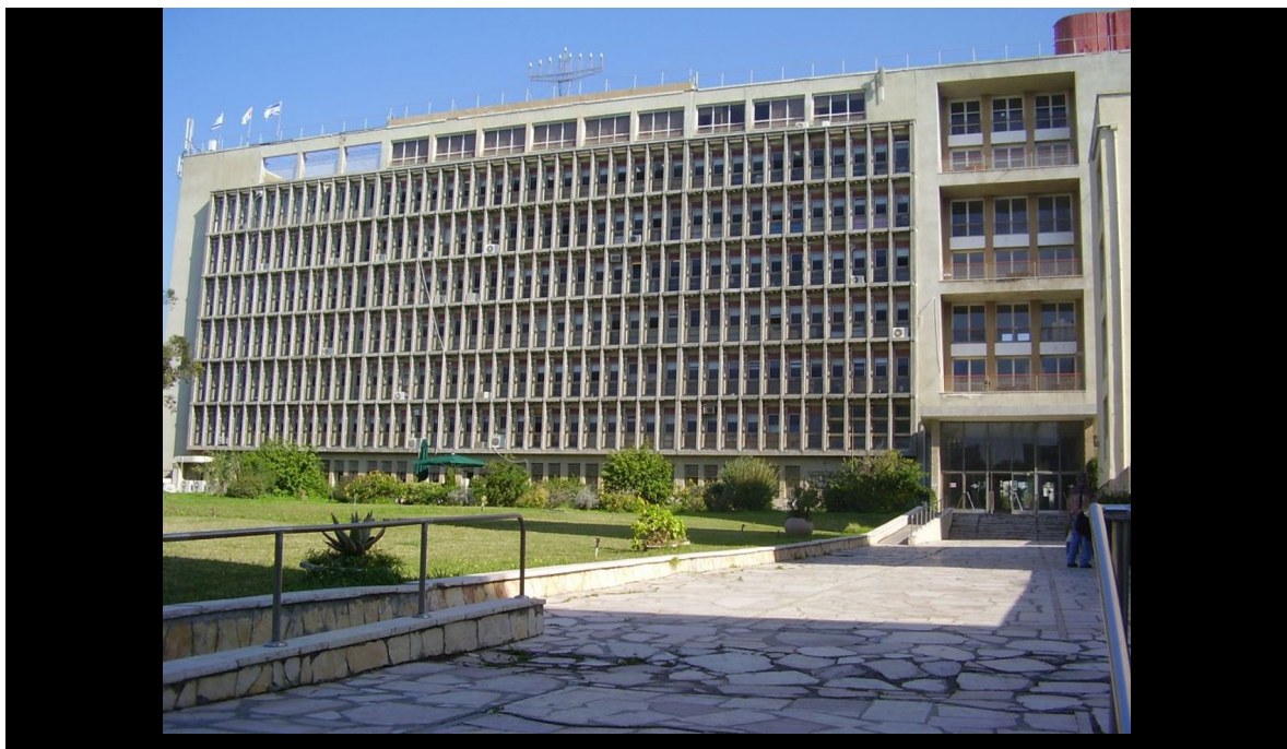
Histadrut headquarters in Tel Aviv [Photo by צילום:ד"ר אבישי טייכר / CC BY 2.5 ]
